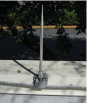
Air terminal screwed to wood nailer Source - FEMA
