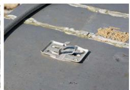
Conductor separated from clip after high wind Source – FEMA
