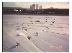
**Roof cover damage from equipment** Source – FEMA
