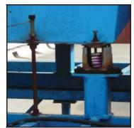
Vibration isolator with threaded rod for upward travel limit
